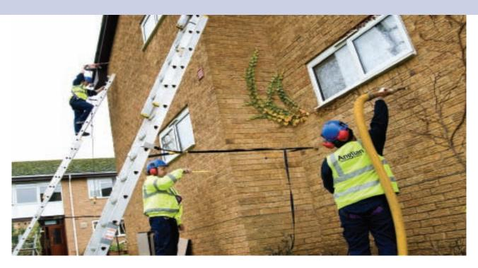
For a traditionally constructed cavity wall property more than a third of all heat can be lost through the walls, therefore insulating the cavity makes obvious sense.
