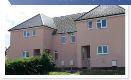
46 residential properties at Lulworth Camp have been fitted with External Wall Insulation to lessen the effect of heat loss through the cavity walled traditional terrace and semi-detached properties.
