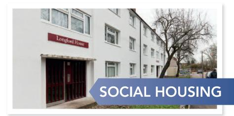
Built in the early 1960's Longford House is a three storey residential block of flats in South West London constructed using the No Fines concrete method.
